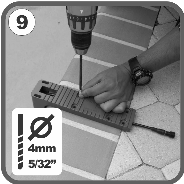
5. Affix the upper hanger directly on the pool edge using hardware kit provided (Fig.9).
